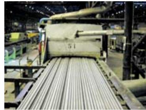
▲ One of the heat-treatment furnaces with an active atmosphere in operation at the Costa Volpino plant.
