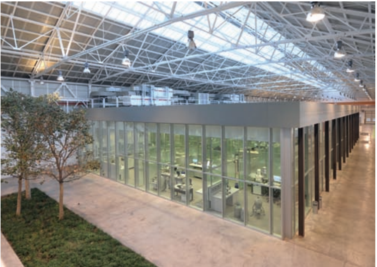
Tenaris R&D Centre in Italy, Dalmine
