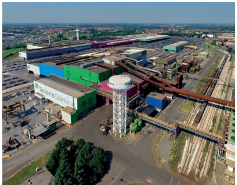
TENARISDALMINE'S STEEL SHOP AERIAL VIEW
