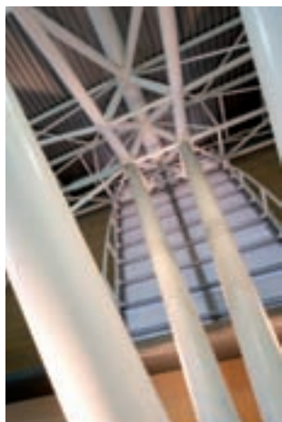
Oval Indoor Stadium, Turin, Italy Bow string truss and supporting structure
