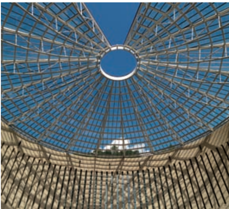
Museum of Modern and Contemporary Art of Trento and Rovereto, Italy / Structure to support the roof
