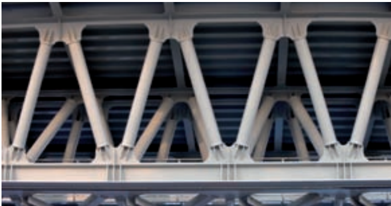
Bridge on the Po river, Piacenza, Italy / Tubular steel supporting the bridge
