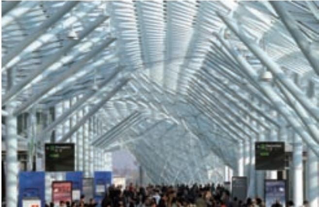
Exhibition center Milan Rho, Italy Structural hollow section to support the "Vela"
