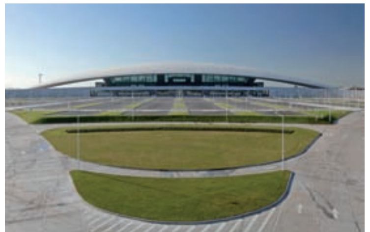
Carrasco International Airport, Montevideo, Uruguay / Supporting structure for roof and glass façade
