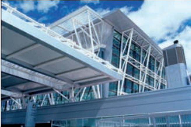
International airport Pistarini, Terminal A , Buenos Aires, Argentina / Canopy roof
