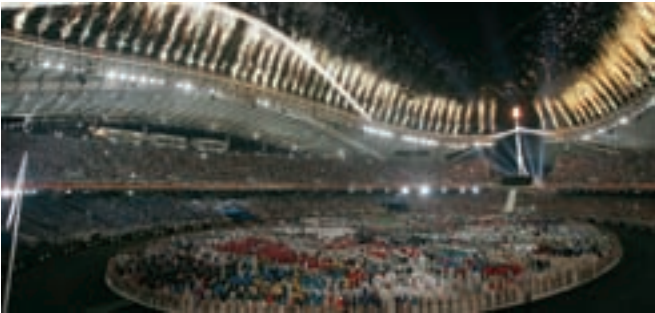
Olympic Stadium Spyros Louis, Athene, Greece / Canopy roof
