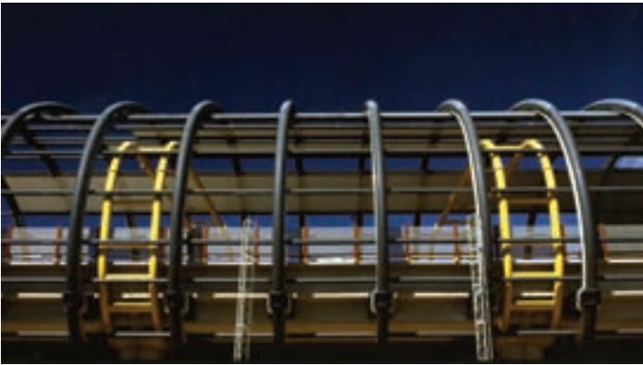
Fiumicino airport, railway terminal, Rome, Italy Circular hollow sections to support the railway
