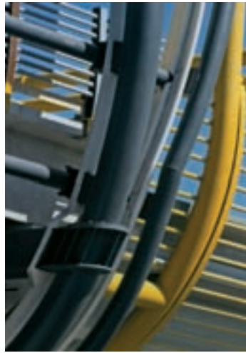
Fiumicino airport, railway terminal, Rome, Italy Circular hollow sections to support the railway
