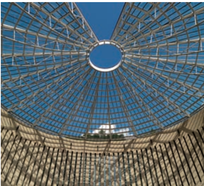
Museum of Modern and Contemporary Art of Trento and Rovereto, Italy / Structure to support the roof
