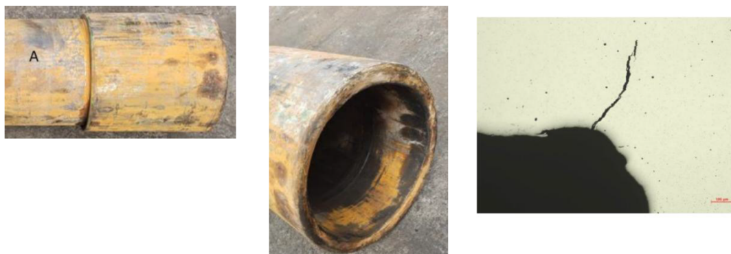
Figure 15—Casing failure. L-4 August 2024.
